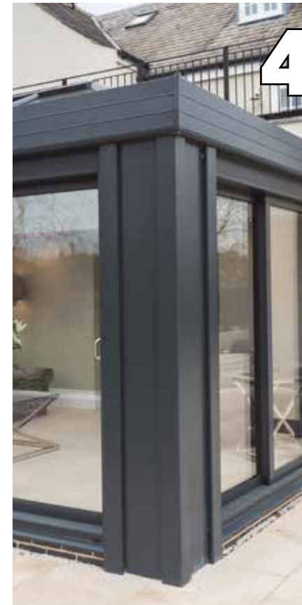
Super-insulated columns and 3 tier flat cornice.
